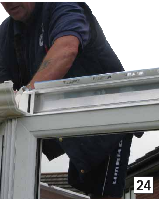
The drainage system will be fitted, including the guttering attached to the eaves beam and any down pipes.
