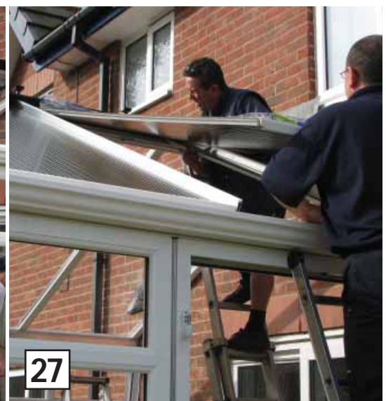
The chosen glazing panels or sealed units are installed.
