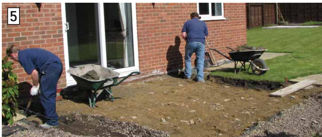
Construction work begins with the digging of the strip footings.
