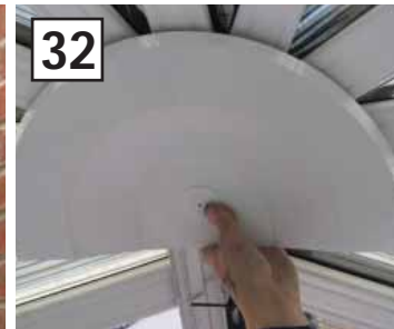
The PVC internal cladding are clipped onto the eaves beam and ridge to complete the internal trims.
