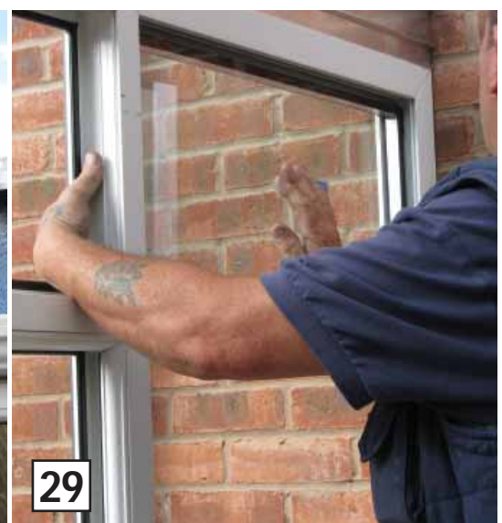
The glazing is installed into the side frames.
