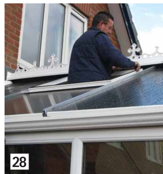
If specified in the plans, a vent will be installed into the conservatory roof.
