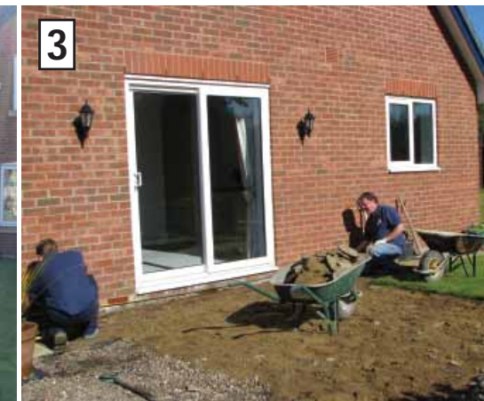
The ground is cleared as part of the preparation process.
