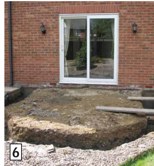
Footings are dug to a minimum depth of 450mm - this will vary depending on the ground conditions.
