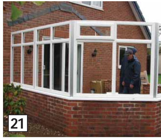
The side frames are 'stitched' together.
