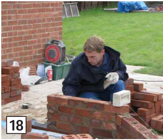
The remaining dwarf walls are built to match the existing brickwork or as requested by the homeowner.
