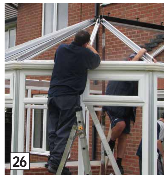
All the glazing bars are fixed from the eaves beam to the ridge.
