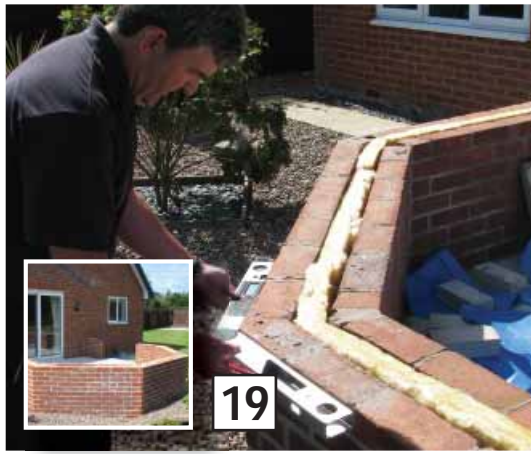
The dwarf walls are built to the height agreed and should include insulation in the cavity wall.
