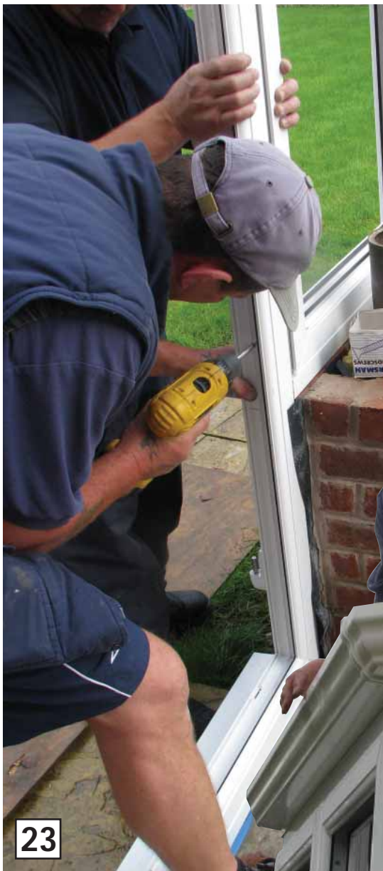
The doorframe is fitted to the side frames and dwarf walls.
