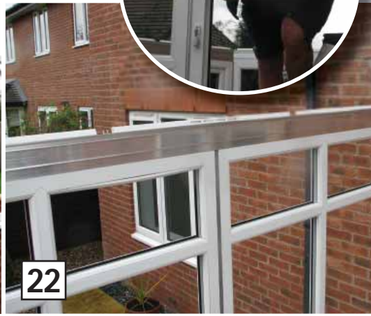
On completion of the frames the structural aluminium eaves beam is fitted to the head of the frames.
