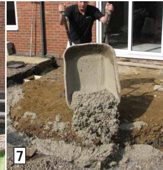
Concrete is poured into the 'trench' to form the foundations.
