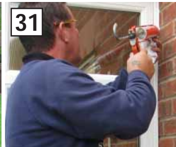
All the finishing touches are added to the conservatory, including the sealing of the side frames against the house wall.
